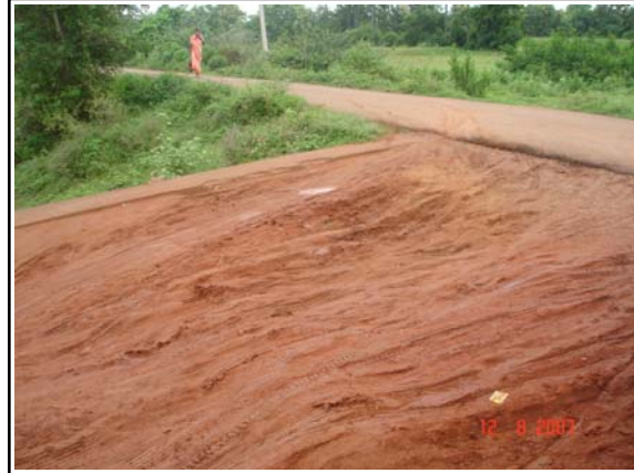
Condition of village roads
