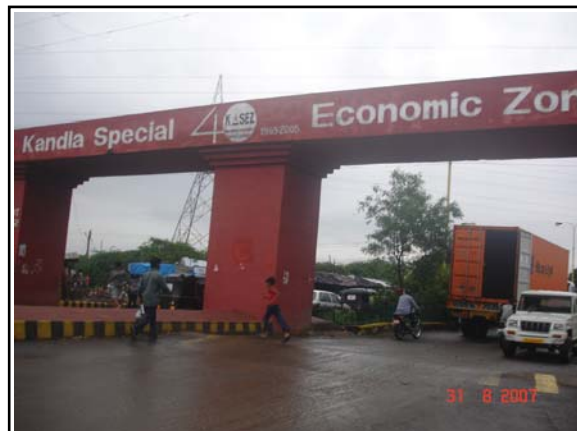
Kandla SEZ Entrance
