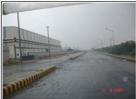
Road inside SEZ
