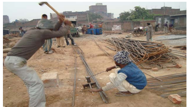
Site of Construction BSUP Phase 3
