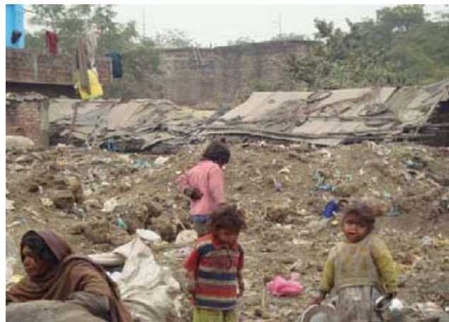
Site of Slum demolition
