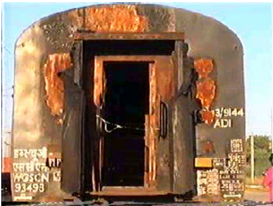
GODHRA COACH, SEAT 72 END. DAMAGE MARKS SHOW FIRE SPREAD TO THE END FROM THE TOP
